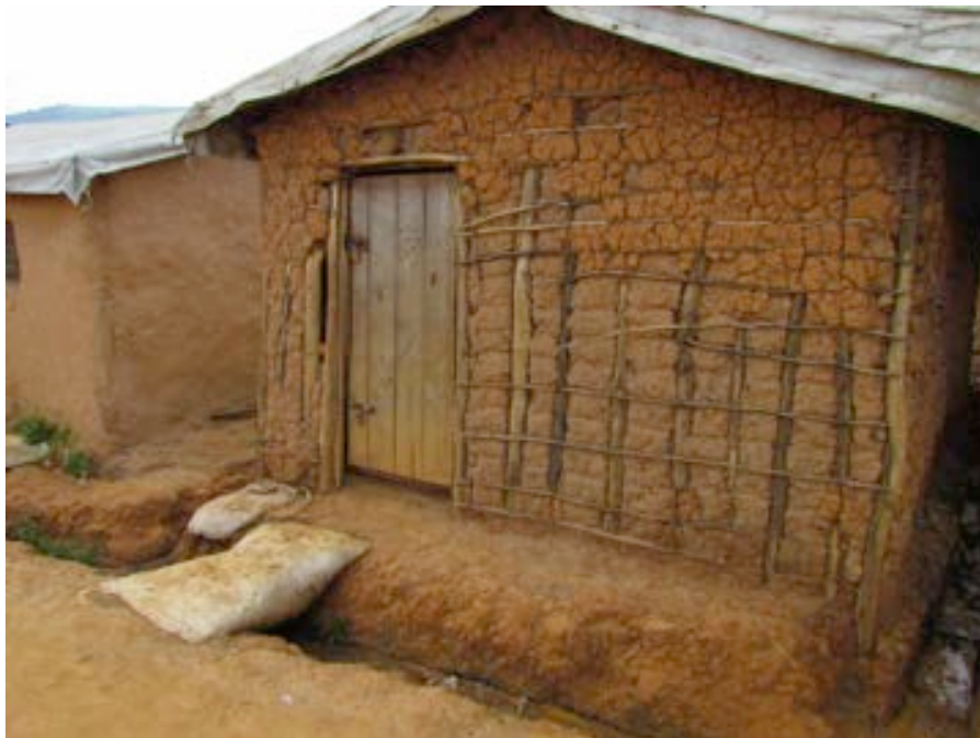
Figure 8: House in Kiziba with scaffolding exposed
