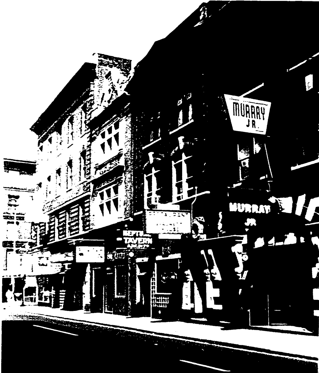
Figure 8. Taverns on Granby Street (120 – 132 block) Murray Jr., Neptune, Royal Palm April 1961 The Murdaugh Collection at Norfolk Public Library
