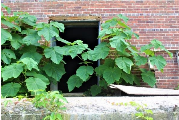
Figure 33. Open entry into the Rosenwald School.
