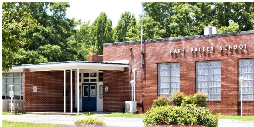
Figure 27. Head Start building.
