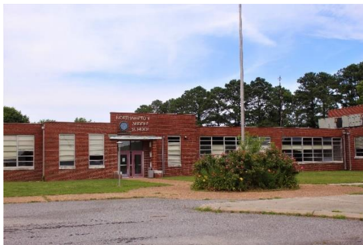
Figure 29. The vacant middle school of Northampton County.
