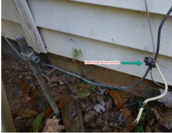
Figure 15: Earth Ground Connection
