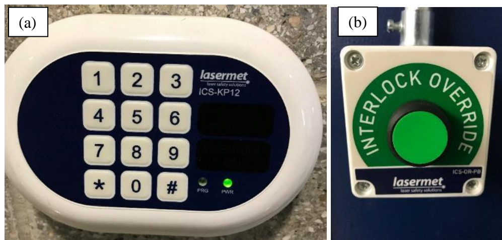
Fig. G.5 (a) Override keypad outside laser lab. (b) override switch inside laser lab. Both are used to temporarily override the laser interlock for 10 sec.
