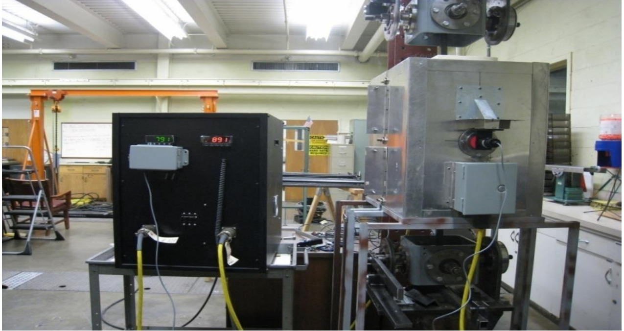
Figure 16. Electric Furnace and Controller
