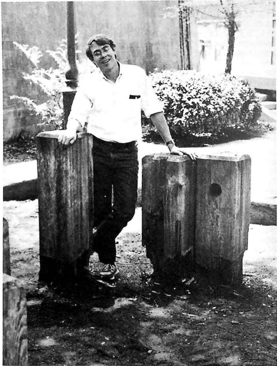
Jeff LaFage in a condemned playground near Jackson Square in the French Quarter of New Orleans, Louisiana, April 27, 1989. He was demonstrating the improper use of untreated wood placed directly into the soil. Photo by Michael Haverty.
